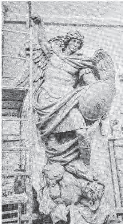
A working model for a statue of St. Michael the Archangel to adorn the facade of Quincy's new police station. Sculptor Sergey Eylanbekov designed the work. Office Of Mayor Thomas Koch
